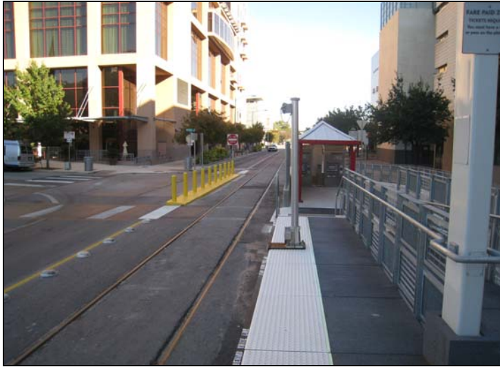
Figure 1-7. Capital Metro Red Line Downtown Terminal Station
